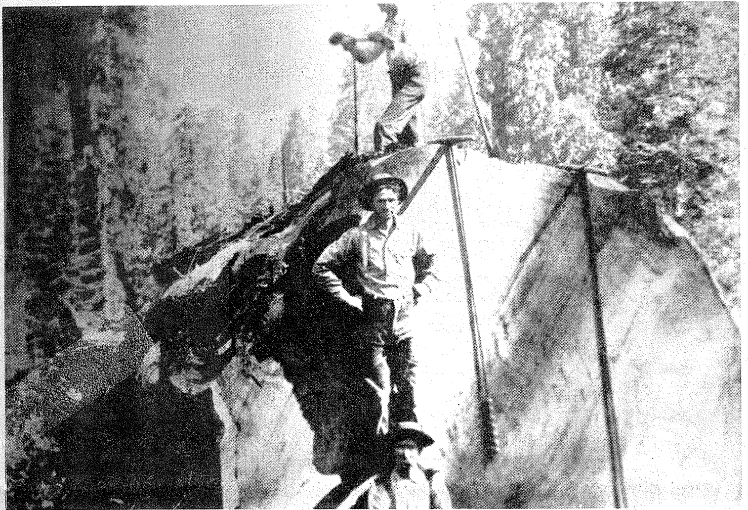
GIANT TREES needed giant augers to drill holes through them so they could be blasted apart with dynamite.
